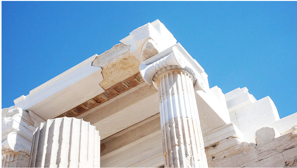
Fig. 4. Acropolis. Propylaea, showing new Ionic column capitals beside central passageway and restored coffered ceiling.
